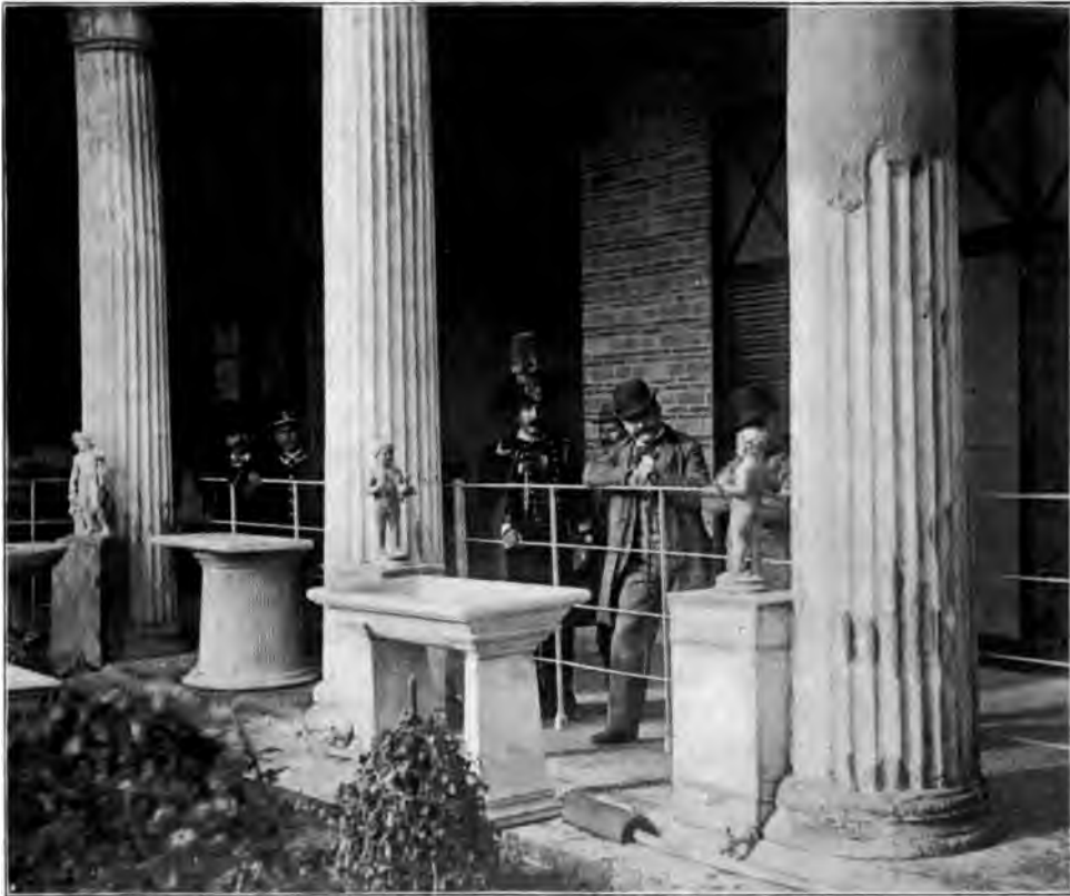
LEAD PIPE, STOP-COCKS, AND FOUNTAIN FIGURES IN THE GARDEN OF THE HOUSE OF VETTI, POMPEII. 2
